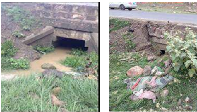
Figure 9a: Culvert Outlet and Inlet
