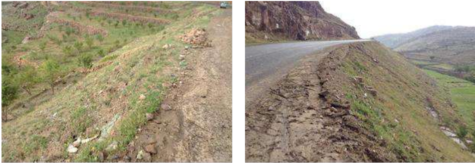
Figure 10a: Water Harvesting from Road Shoulders
