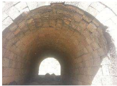
Figure 4b: Arched Stone Culverts
