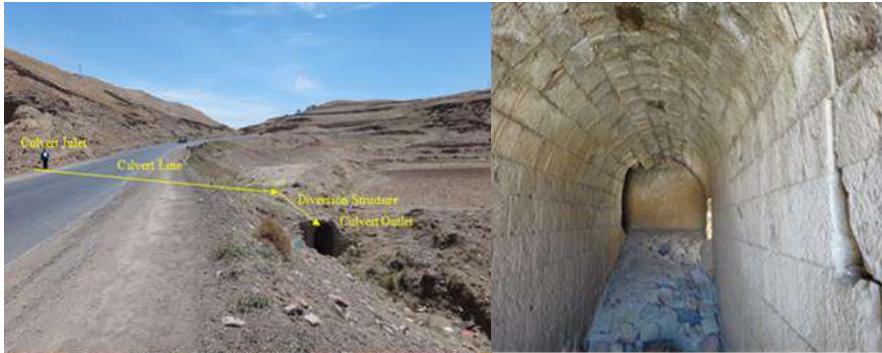
Figure 6: Culvert with Right Angle Direction, Used as Diversion Structure
