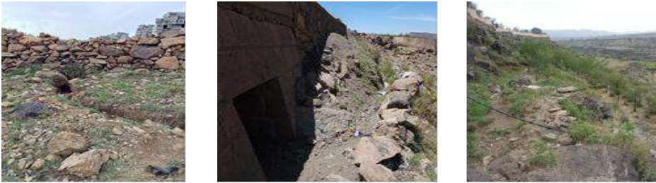
Figure 8: Harvested Water from Culvert by Earthen Canal to Almond Farm
