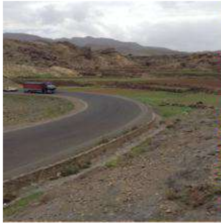
Figure 5a: Side Ditch
