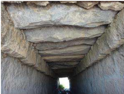
Figure 4a: Girder Stone Slab Culverts
